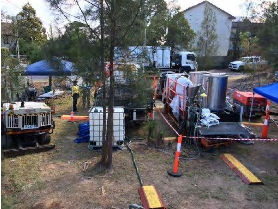
Photo 4 – Example Injection of Oxidant
