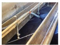
Granular Activated Carbon (GAC) is removed from each of our 26 filters every three years and regenerated carbon is put back in the filter through a hose as shown here (see above).
