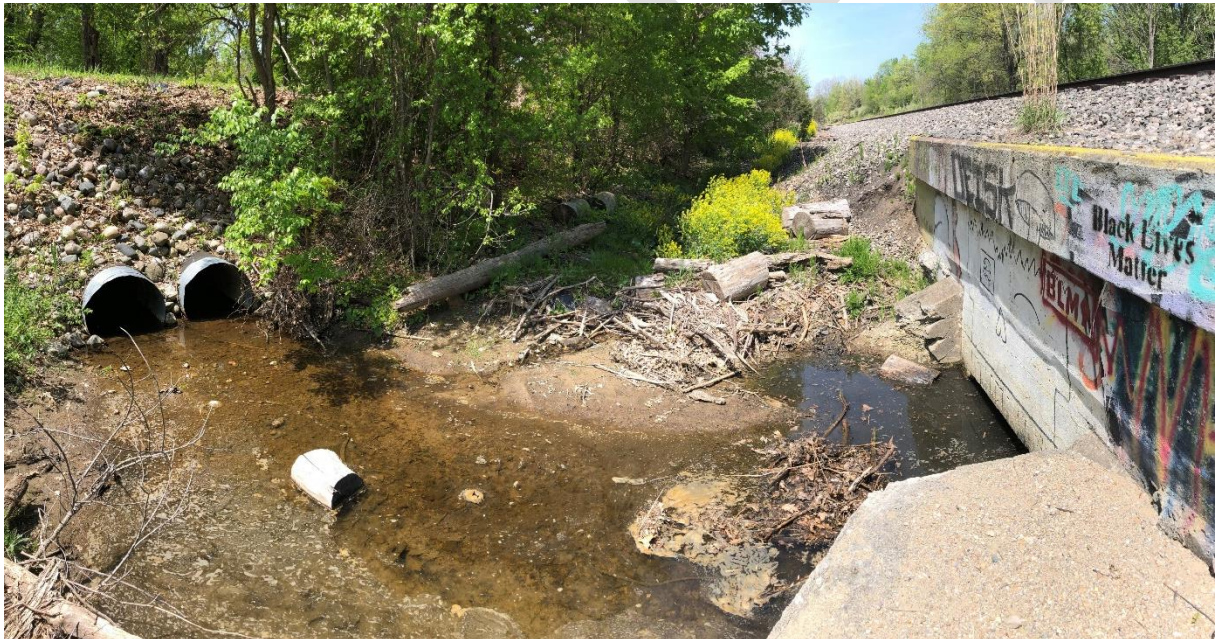
Figure 17. Floodplain culverts set at a higher elevation for flood flows.
