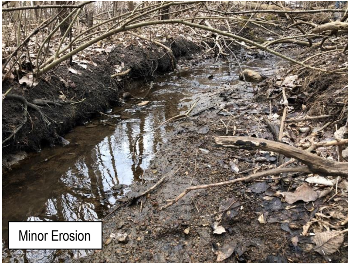
Figure 2. Examples of erosion severity seen along Newport Creek.
