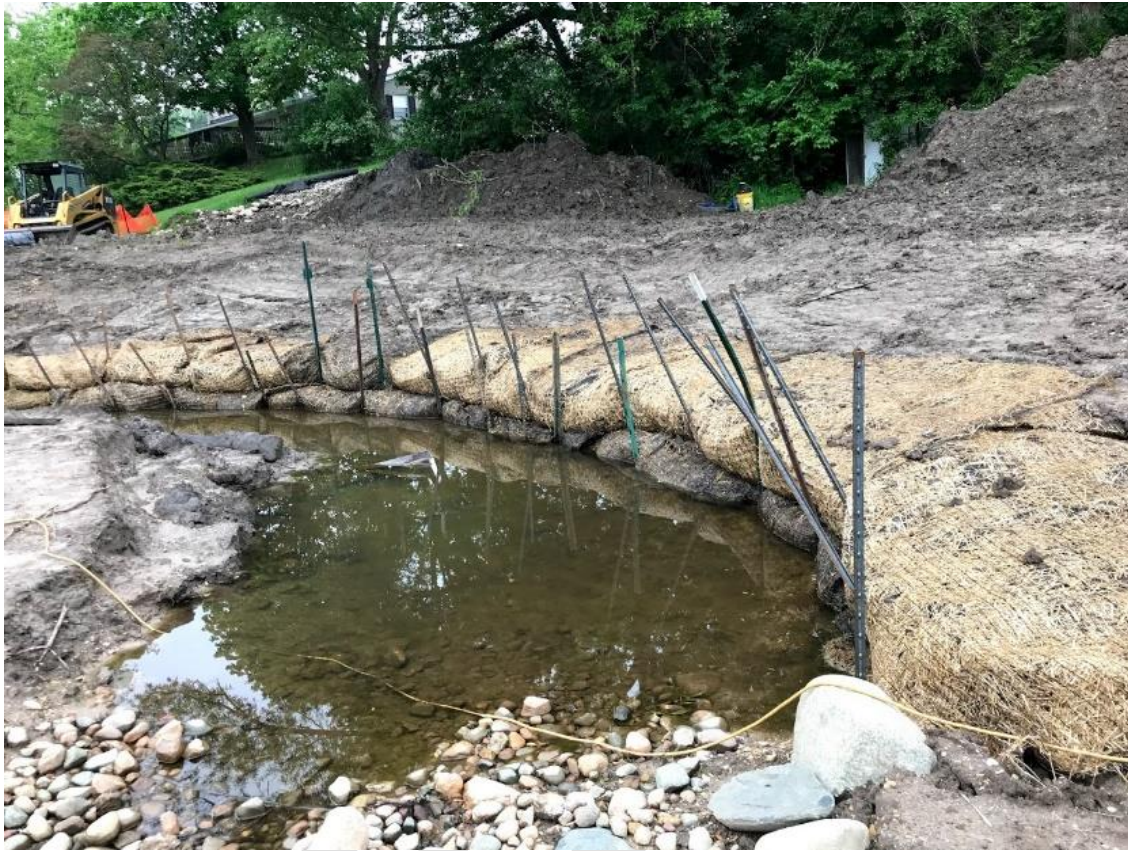
Figure 15. Vegetated reinforced soil slope system (VRSS).
