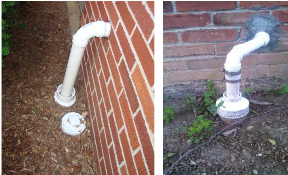
Photo 3 & 4 – Original (2001 – 2011) Air Gap Configurations
