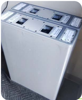
16 kW of battery storage that was installed at Creekside Commons.
