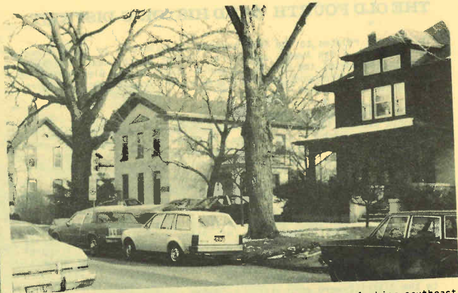
5-600 block of Lawrence Street, looking southeast.
