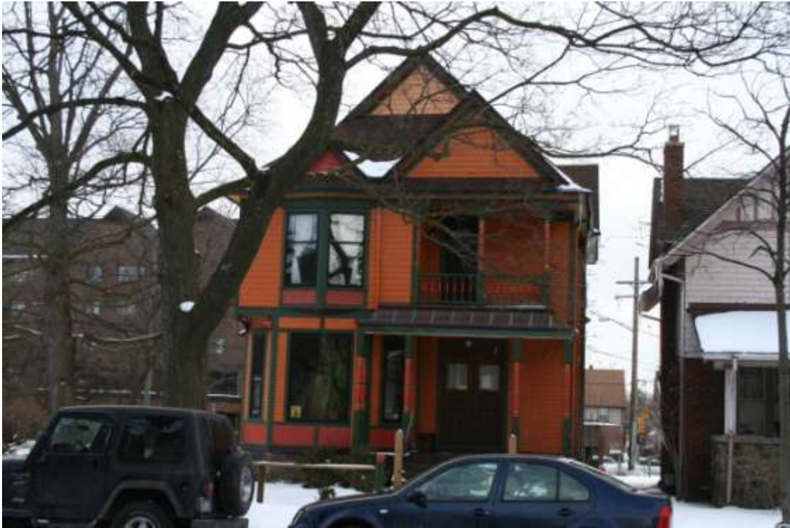
Photograph 12 – 442 South Fourth Avenue, Gottlieb Wild house, February 2010
