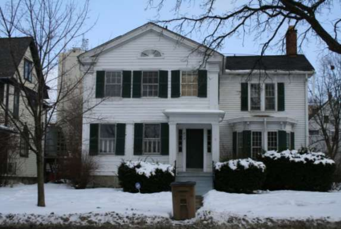
Photograph 6 – 415 South Fifth Avenue, Gaskell/Beakes House, February 2010
