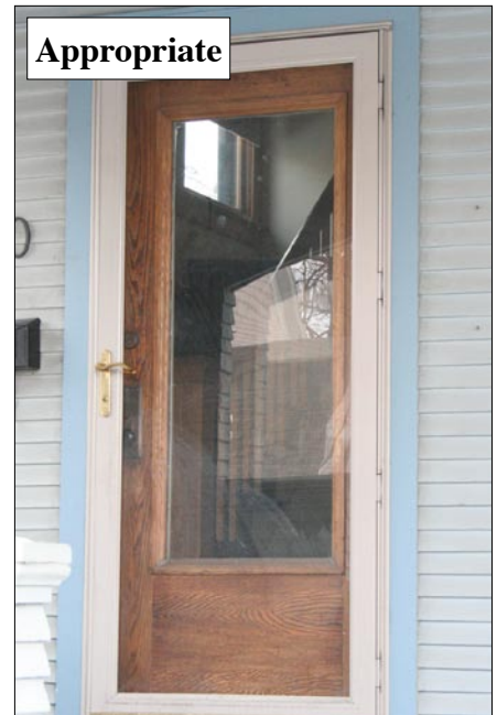
Retain, repair and maintain original doors.
