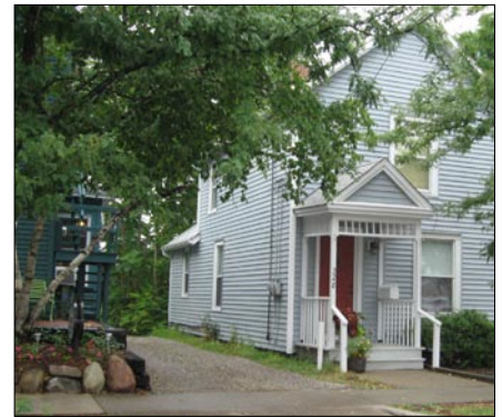
Additions to historic residential structures should be inconspicuous and should not compromise the historic integrity of the original structure.
