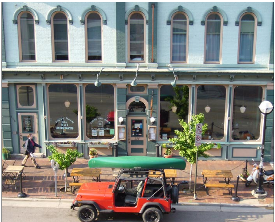
The storefront is the most prominent feature of most historic commercial buildings.
