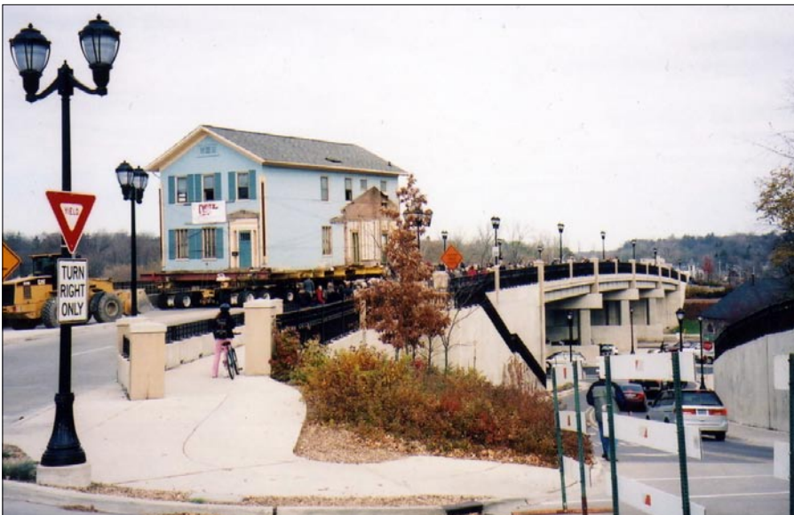
Although moving a building that contributes to the character of a historic district should be avoided, it may occasionally be appropriate to do so in order to avoid demolition.
