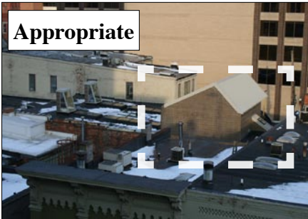
Rooftop additions to commercial buildings should be as inconspicuous as possible when viewed from the street.
