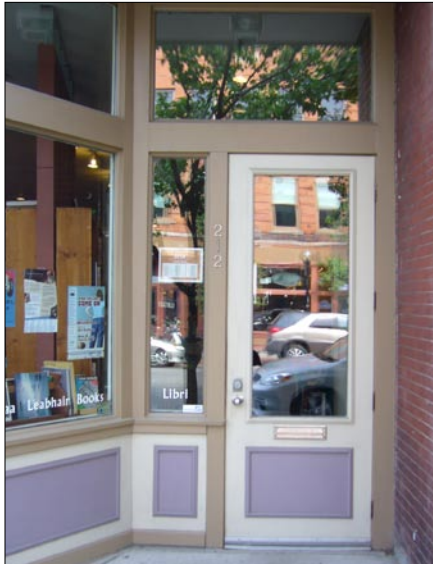
Retain, repair and maintain original doors and trim including surrounds and transoms.
