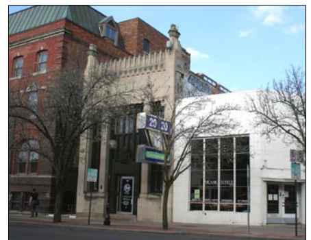
While a number of general principles apply to all new construction in historic districts, some principles depend on whether the construction is within a historic residential or commercial setting.
