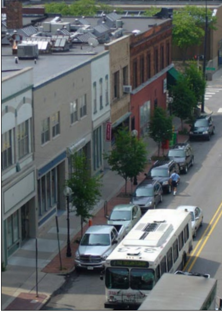
Historic commercial buildings such as those in the Main Street Historic District usually have flat roofs.
