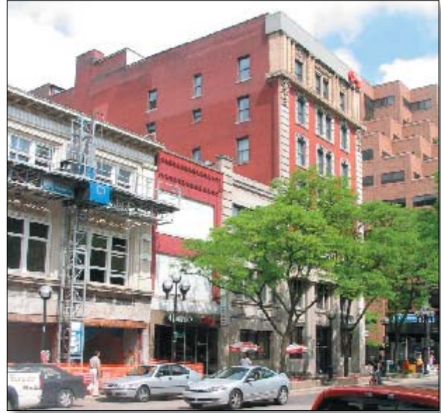
Fig. 1. Main Street Mixed Use Area
