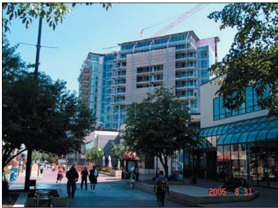
New Construction - Iowa City
