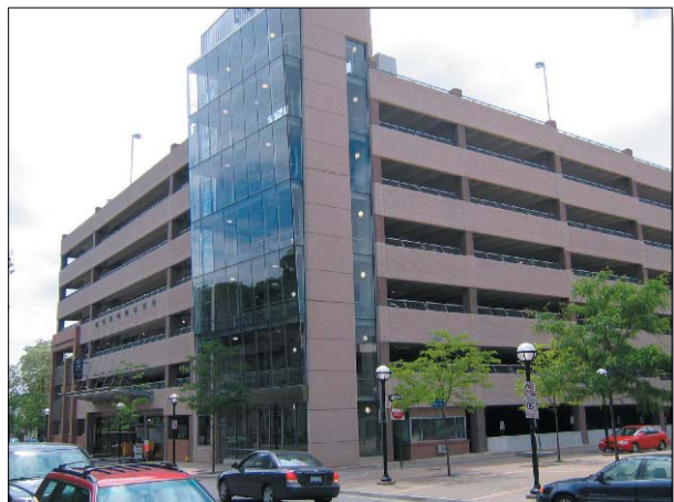
Fig. 43. Forest Street Parking Garage
