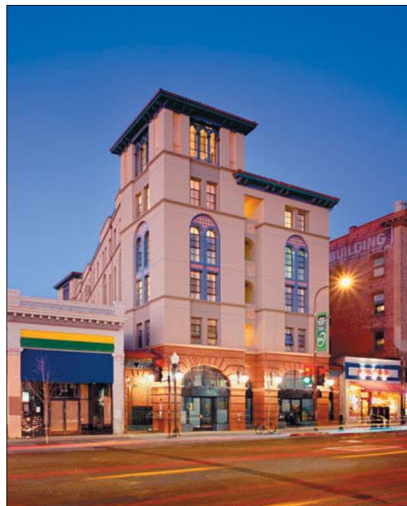
Bachenheimer Building - Berkeley
