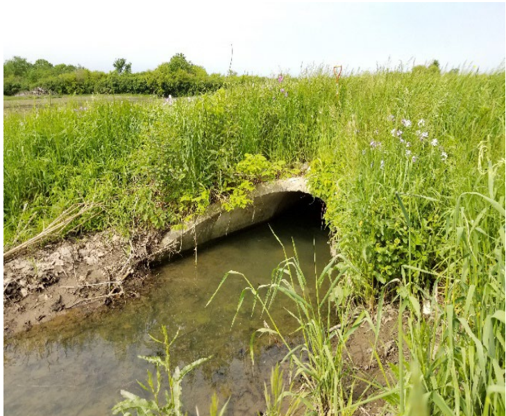
Culvert for the Unnamed Drain
