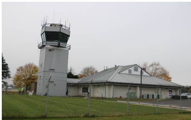
Airport Traffic Control Tower
