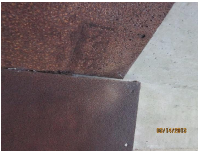
Photo 3 Station 100+45: steel reinforcement
