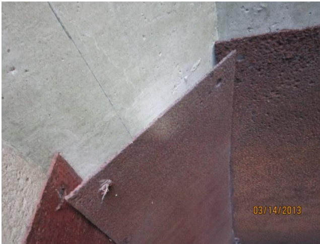
Photo 2 Station 100+45: steel reinforcement
