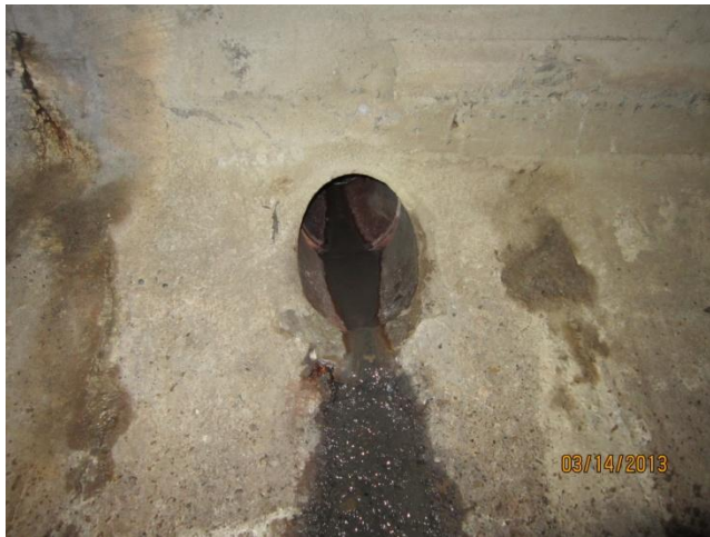
Photo 29 Station 700+65: 12" clay pipe, good
