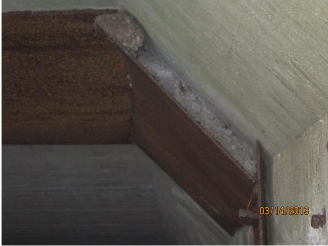
Photo 1 Station 100+45: steel reinforcement
