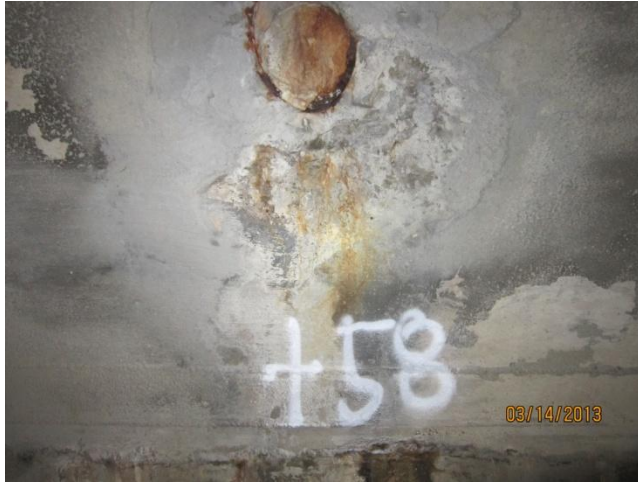
Photo 28 Station 700+58: 6" bulk head, good
