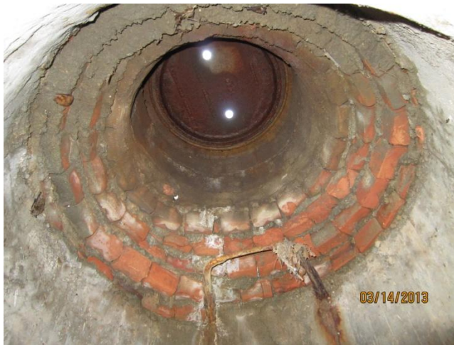
Photo 32 Station 800+20: manhole #2, good condition
