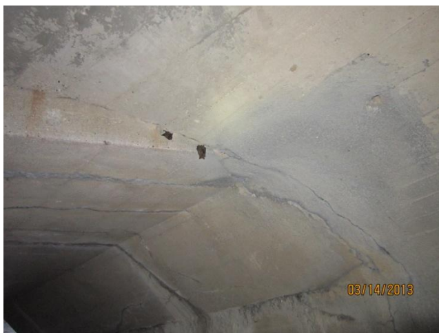
Photo 6 Station 100+90: pipe transition, good
