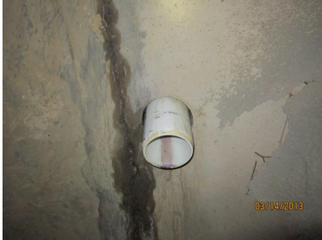
Photo 19 Station 300+80: 6" PVC pipe, good condition
