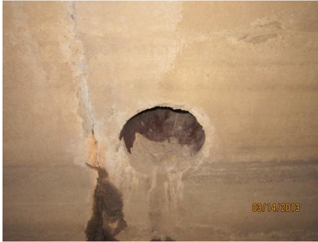
Photo 10 Station 200+82: 12" clay pipe, good
