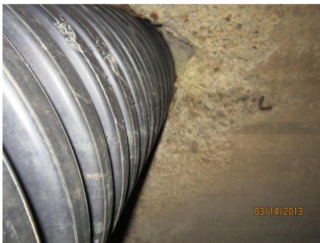
Photo 12 Station 200+95: 12" HDPE pipe, good
