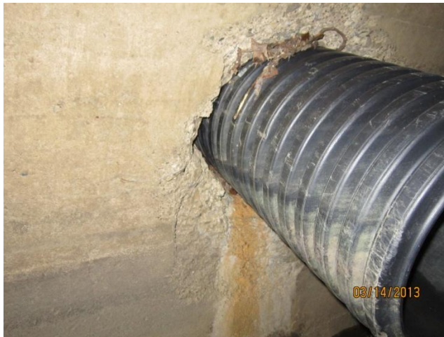
Photo 11 Station 200+95: 12" HDPE pipe, good
