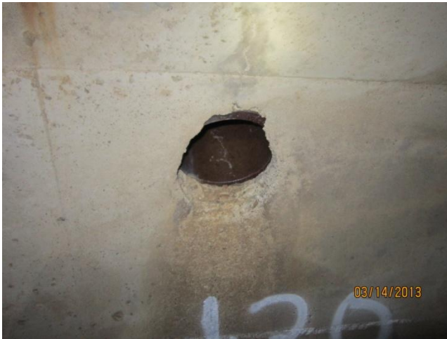
Photo 26 Station 600+30: 4" clay pipe, good
