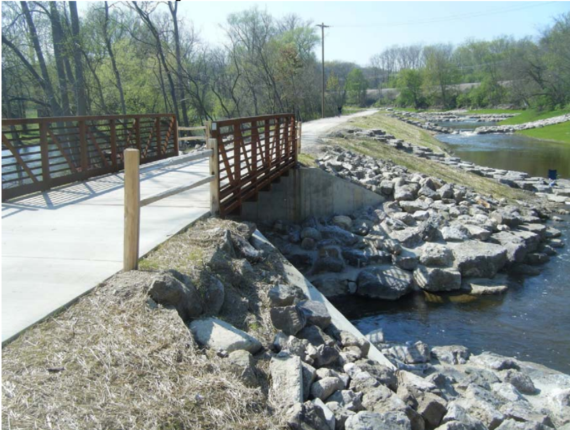
Exit Bridge; north side, facing west
