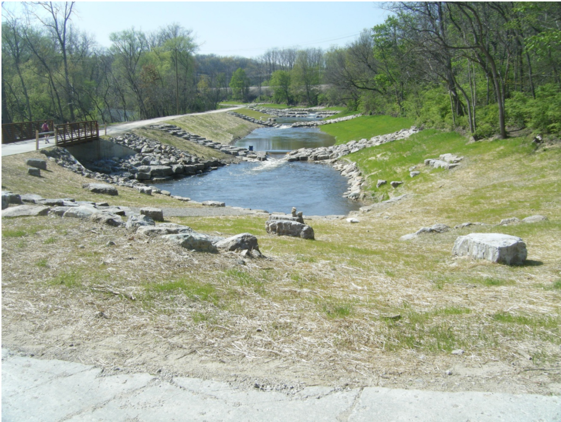
Riverbank at Cascade's toe and Exit Bridge, from hilltop; facing west
