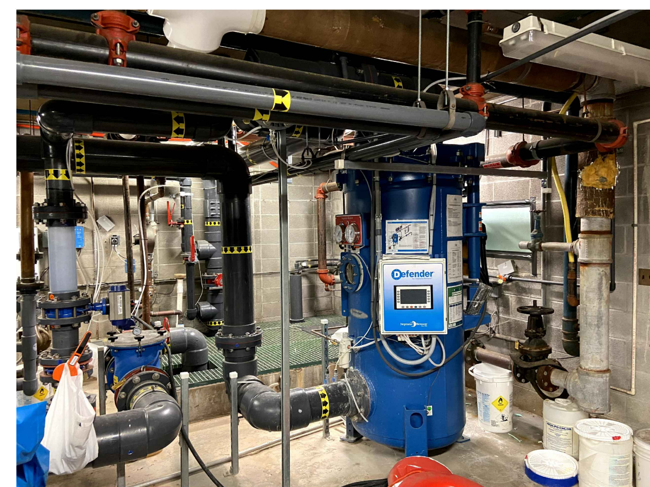
EXISTING POOL FILTER PIPING
