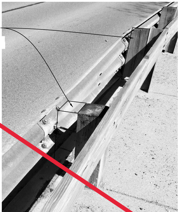
OFFSET BLOCK REPLACEMENT DETAIL
