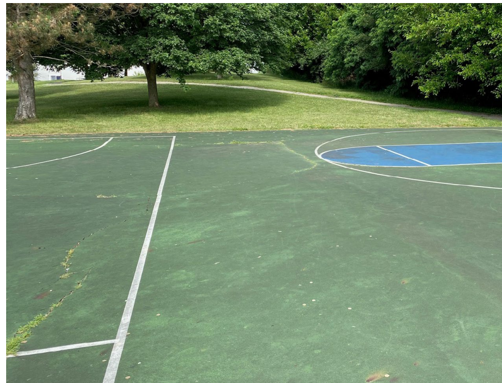
EXISTING SURFACE CONDITION
