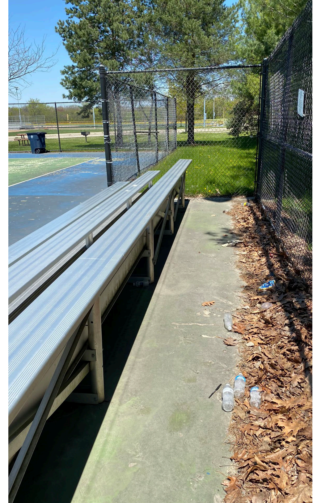
ALUMINUM BLEACHER WILL NEED TO BE REMOVED DURING CONSTRUCTION AND REINSTALLED AFTER.
