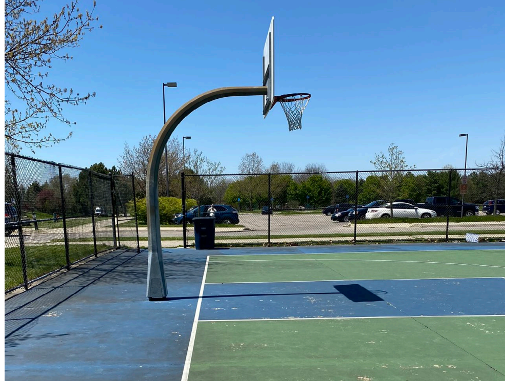
BASKETBALL EQUIPMENT (POLE FOUNDATION, POLE, BACKBOARD, RIM) TO REMAIN DURING CONSTRUCTION
