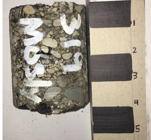
319 Mosley Street in Eastbound Lane
