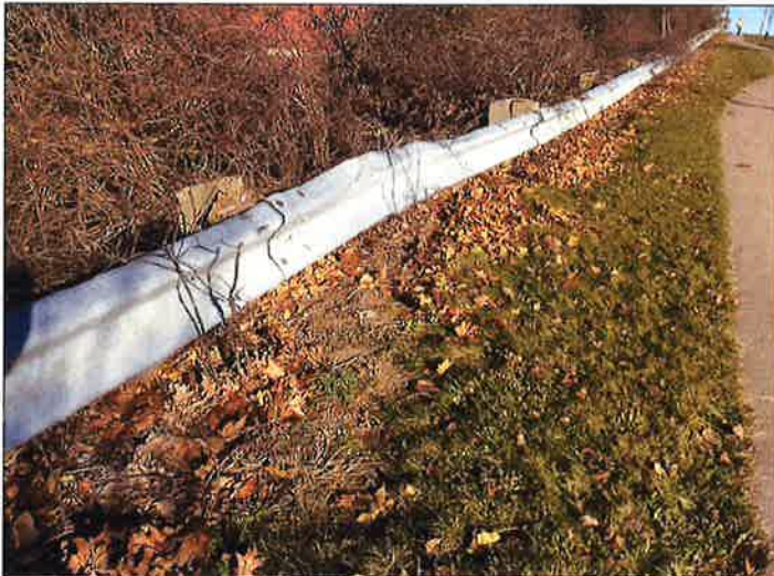
Defect 1: Guardrail damage
