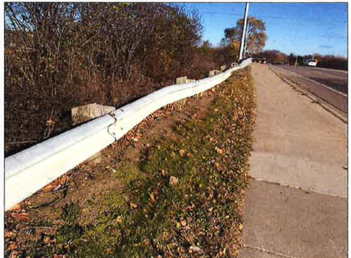
Defect 2: Guardrail damage
