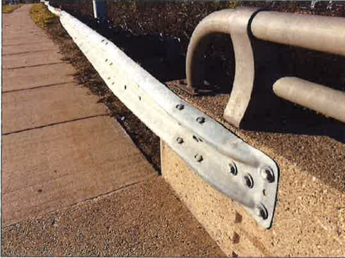
Defect 1: Guardrail damage
