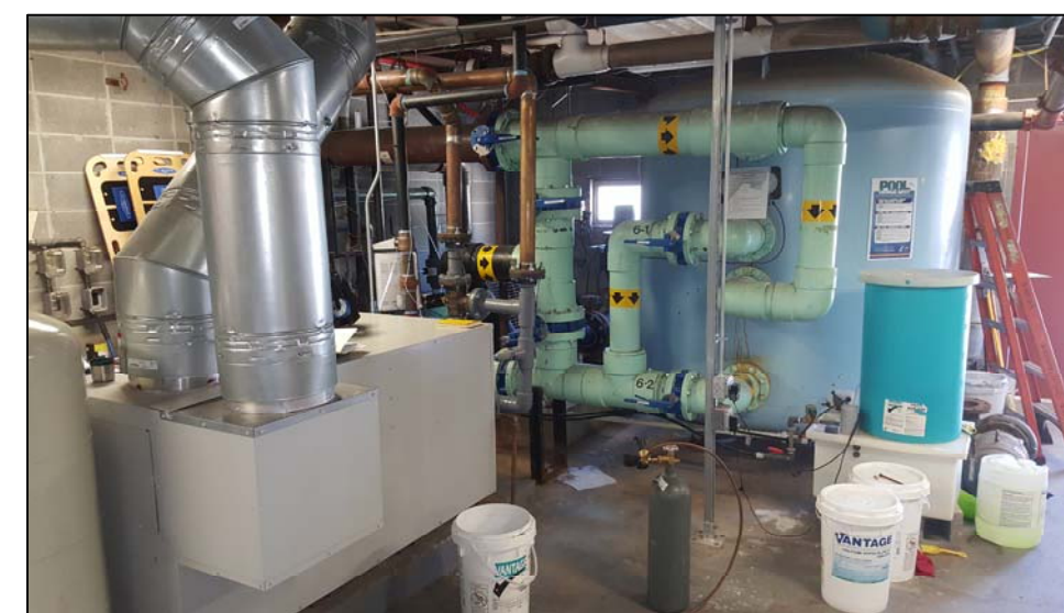
EXISTING FILTRATION SYSTEM & PIPING TO BE DEMOLISHED
