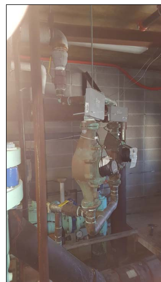
EXISTING WATER METERS TO BE RELOCATED
