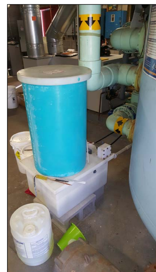
EXISTING VANTAGE FEEDER TO BE SALVAGED & RE-INSTALLED
