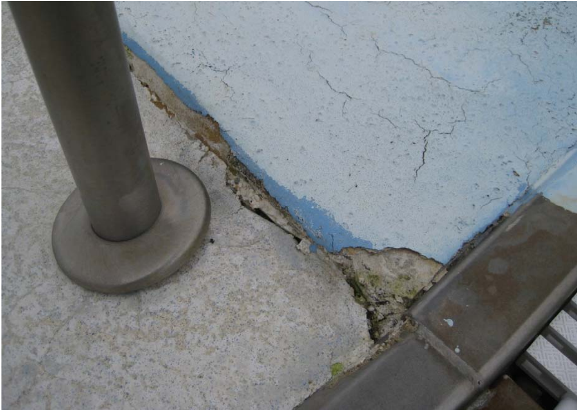
Spalling concrete
