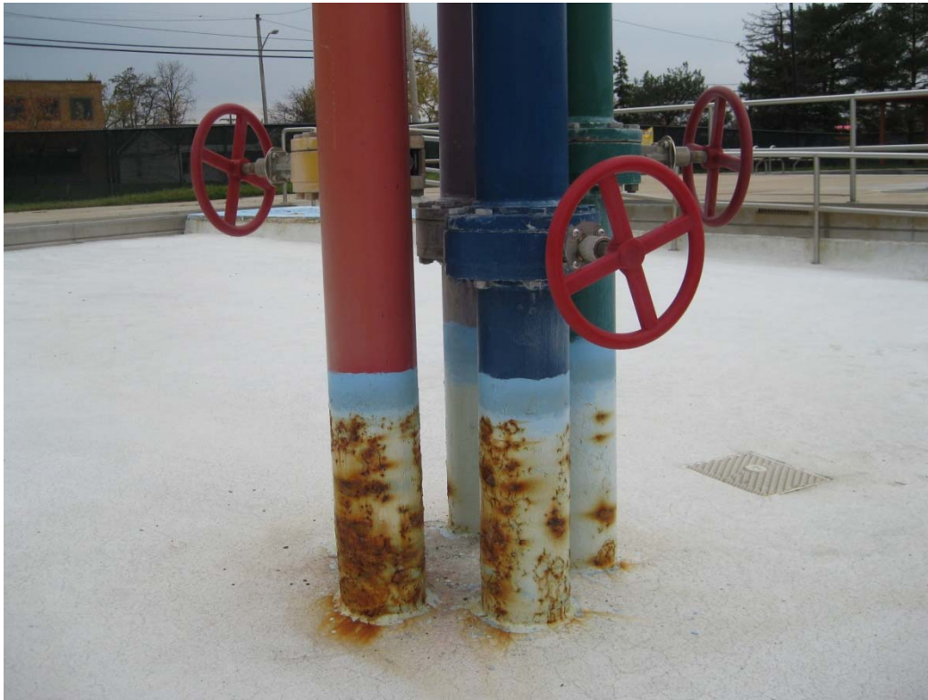
Base condition of water feature in wading pool
