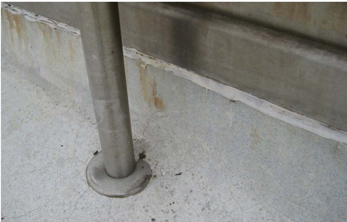
Install base cones on handrail system
