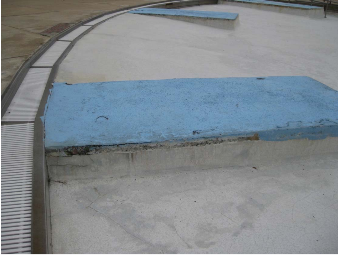
Concrete pads in wading pool
