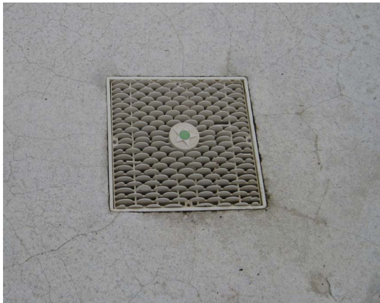
Grate in wading pool
