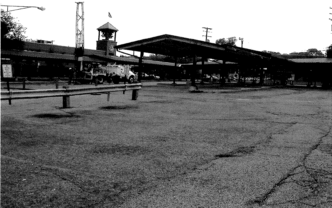
Photograph No. 2 From Boring B-6, facing northeast.
