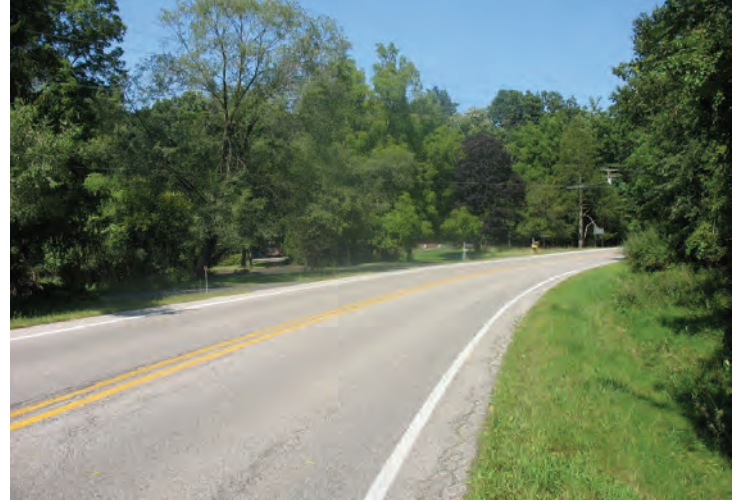
Facing north from the southwest portion of the Subject Property viewing the north adjacent property. North Wagner Road is observed in the foreground.
