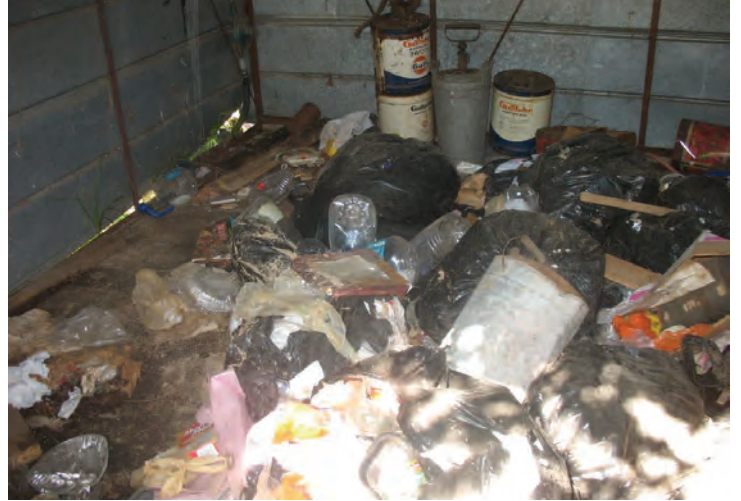
Viewing the interior of the storage shed.
