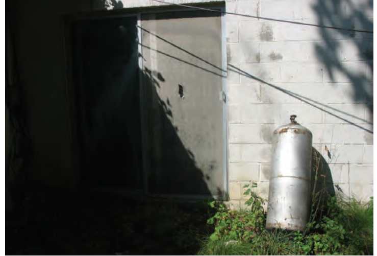
Facing north viewing an approximate 100 gallon propane AST located adjacent to the house.
