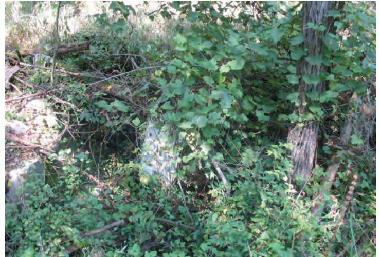
Viewing the remnants of a building foundation and a washing machine located in the southeast corner of the Subject Property, adjacent to the aforementioned potential vent pipe.
