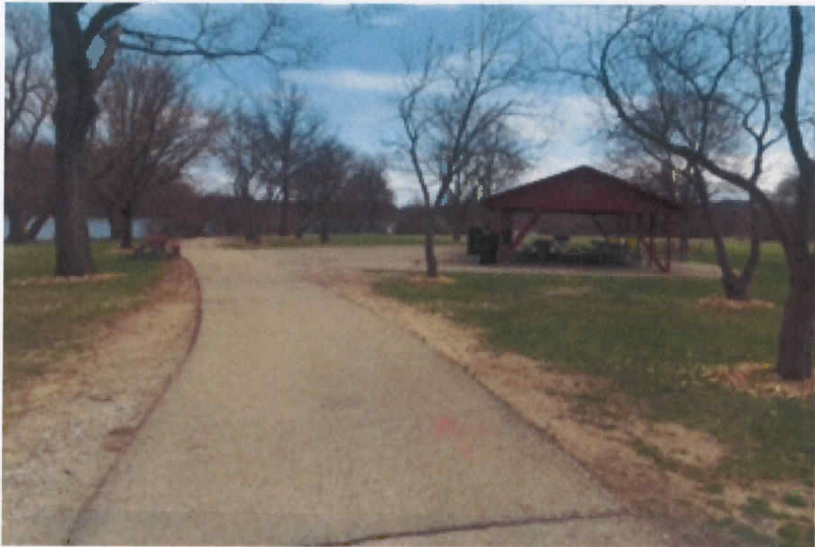
Existing Picnic Shelter to be replaced
