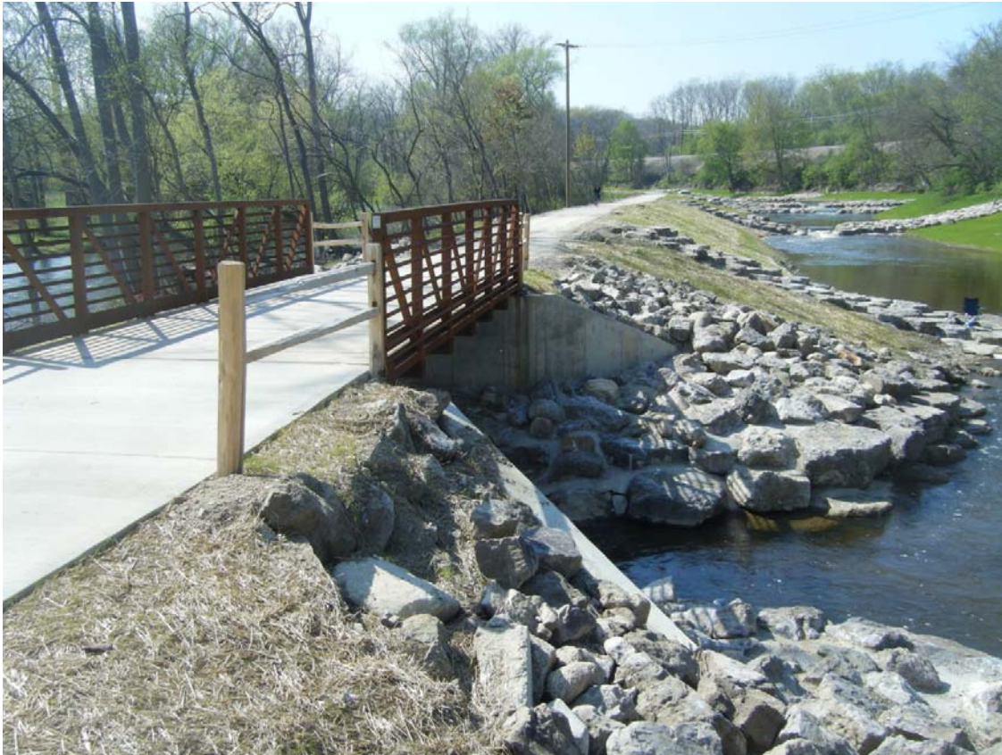
Exit Bridge; north side, facing west
