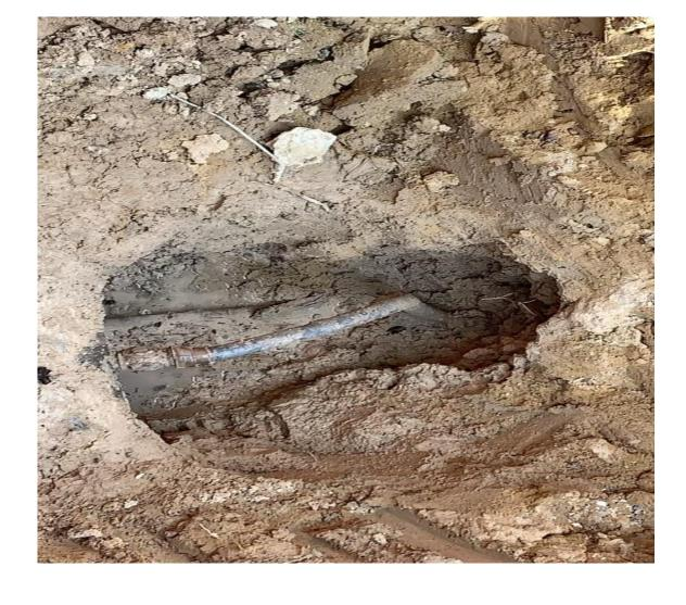
**Galvanized Water Line Replacements:** Federal and State legislation requires utilities to remove galvanized water service leads where they have been in contact with sources of lead. Ann Arbor estimates that it has approximately 1000 of these service leads remaining in its system that will need to be replaced. Expedited removal of these service leads will remove a known public health risk.
