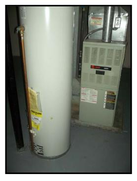
PHOTOGRAPH NO. 9: TYPICAL VIEW OF HOT WATER HEATERS AND FURNACES IN TENANT UNITS
