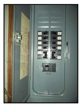
PHOTOGRAPH NO. 7: TYPICAL VIEW OF ELECTRICAL PANELS IN TENANT UNITS
