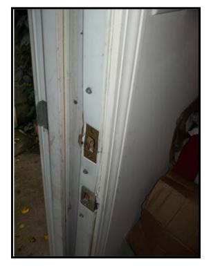
PHOTOGRAPH NO. 18: VIEW OF DAMAGED DOOR FRAME IN TENANT UNIT 241
