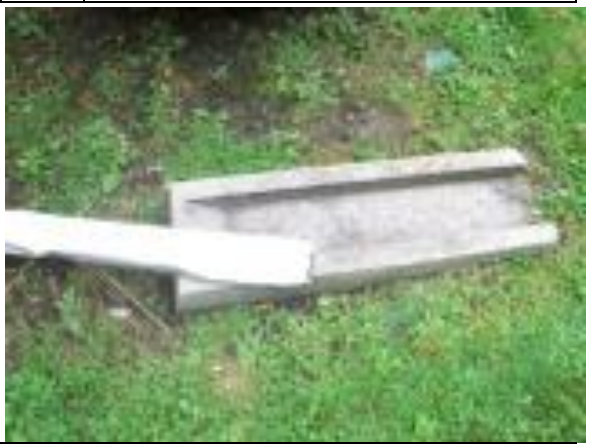
Photo #18: Water pool here if not adjusted.
