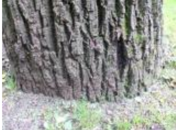
Photo #10: Tree with damage close to building has ants. Branches overhanging should be trimmed.
