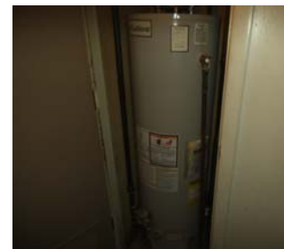
Existing tank at sample unit > 20 years old
