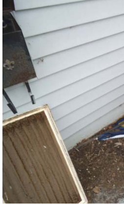
Photo 7: Older furnace filter
