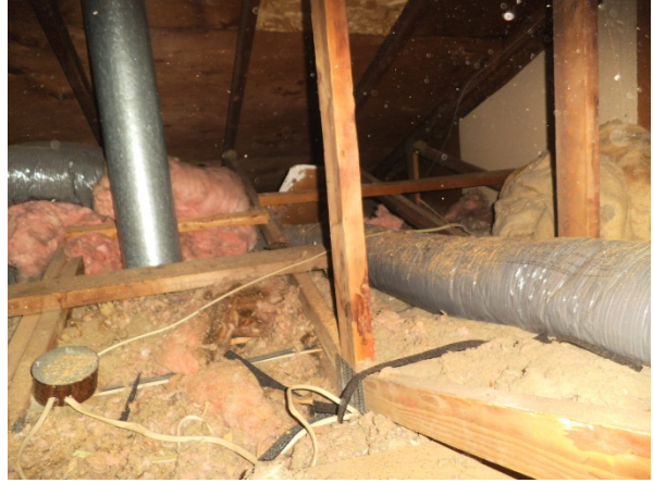
Photo 14: Blown insulation in attic space
