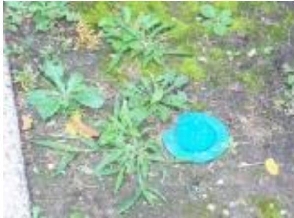
Photo #2: Location previously had issue with termites. Termite stations.
