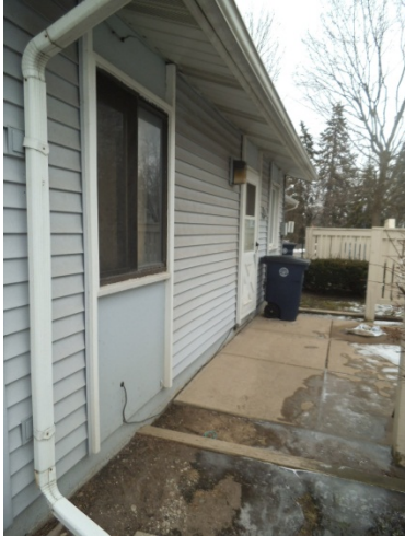
Photo 1: Front view of complex
