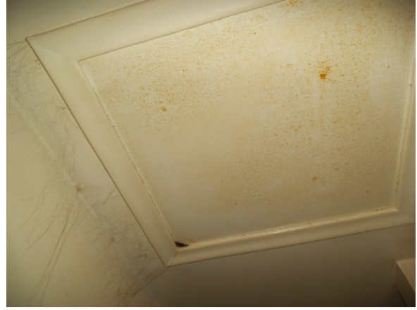
Photo 16: Hatch to attic space
