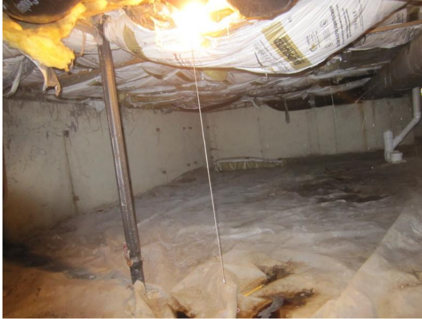
PHOTOGRAPH NO. 13: TYPICAL VIEW OF CRAWL SPACE
