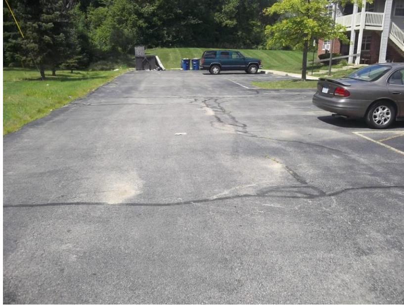
PHOTOGRAPH NO. 5: SECOND VIEW OF PARKING LOT
