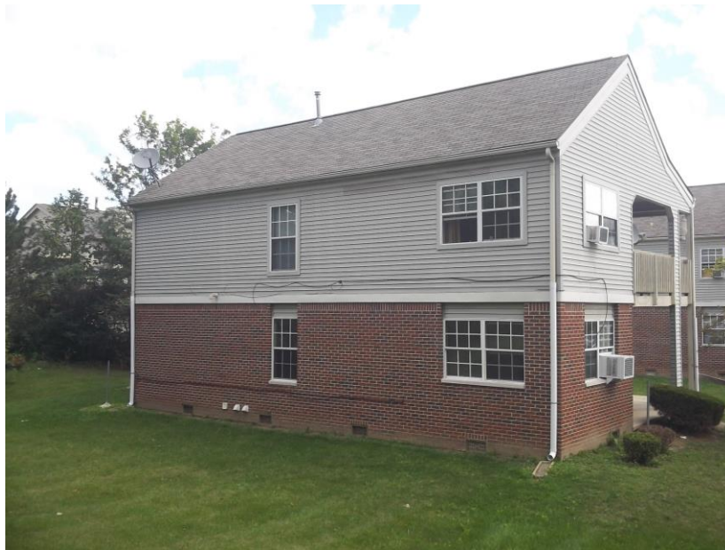
PHOTOGRAPH NO. 2: TYPICAL VIEW OF SIDE OF TENANT BUILDING
