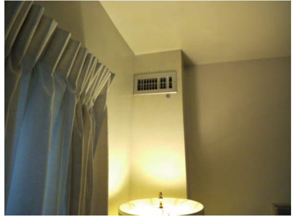
Photo 38: Supply register for fan coil unit in wall
