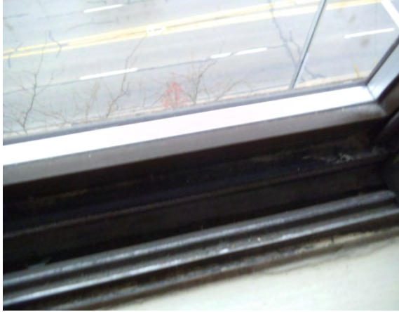
Photo 37: Window frame in fifth floor units
