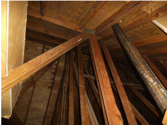
Photo 33: Framing for attic space
