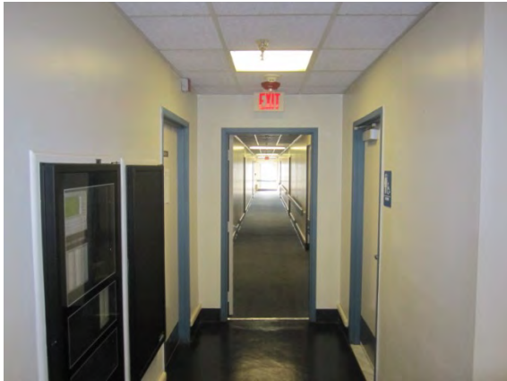
Photo 19: First floor hallway near common area
