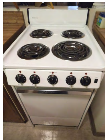
Photo 36: Typical electric stove in apartments
