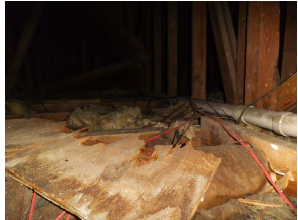
Photo 32: Attic space above fifth floor
