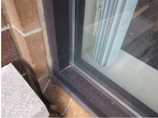
Photo 7: Window frame of first floor windows
