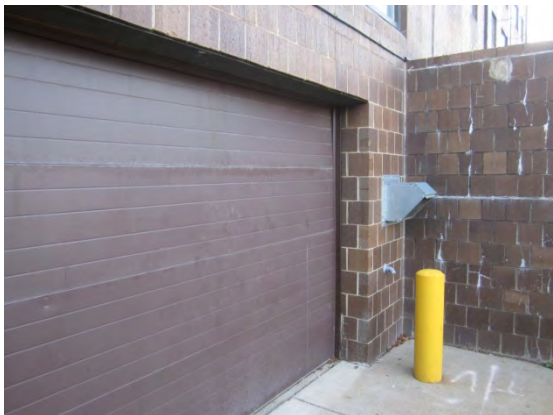
Photo 11: Overhead garage door for basement
