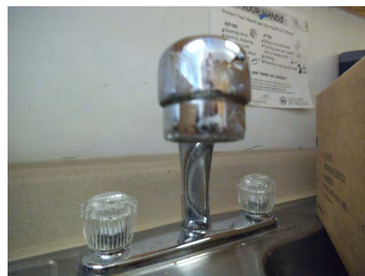
Photo 30: Common area kitchen sink faucet
