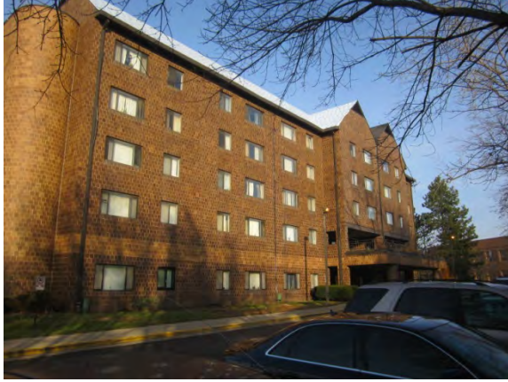
Photo 1: Parking lot view of complex
