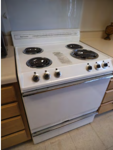
Photo 31: Common area kitchen electric stove
