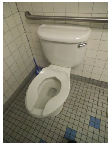
Photo 28: ADA accessible common area bathroom
