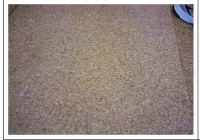
**Photo 6.** View of the asbestoscontaining linoleum pebble pattern
