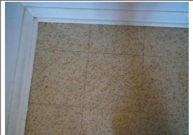
**Photo 5.** View of the asbestoscontaining 9" x 9" floor tile
