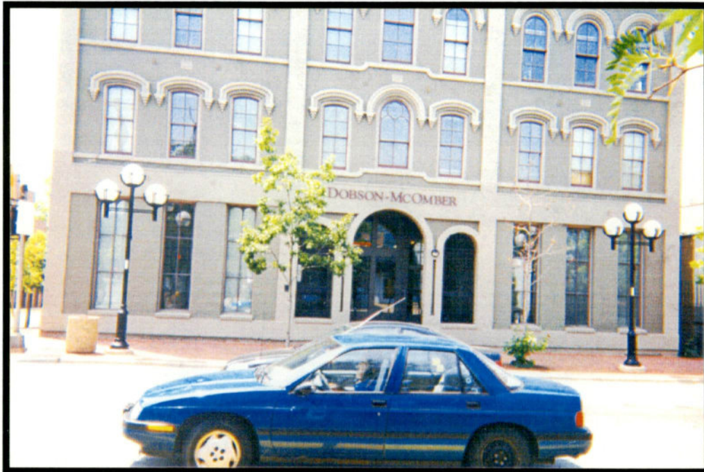
Photograph No. 3 Adjoining Property: East Beyond North Main Street Multi-tenant Commercial Development
