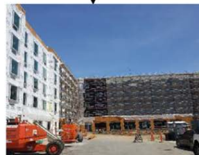
4. Siding & Roofing Outside, MEP & Finish Inside
