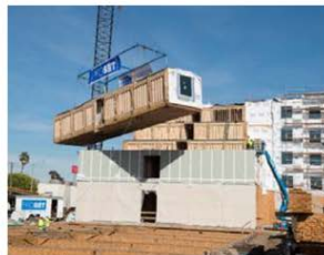
3. Craned and Connected
