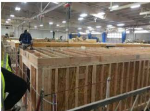
1. Modules Built in Factory
