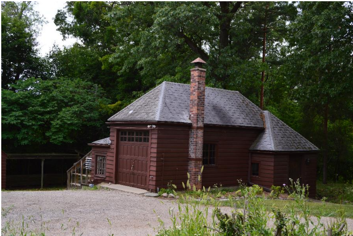
6 - Looking southwest at shop and greenhouse, July 2017
