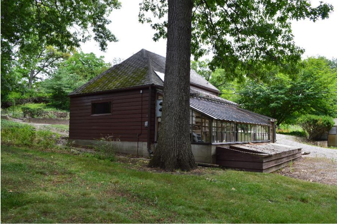
7 - Looking northeast at shop and greenhouse, July 2017
