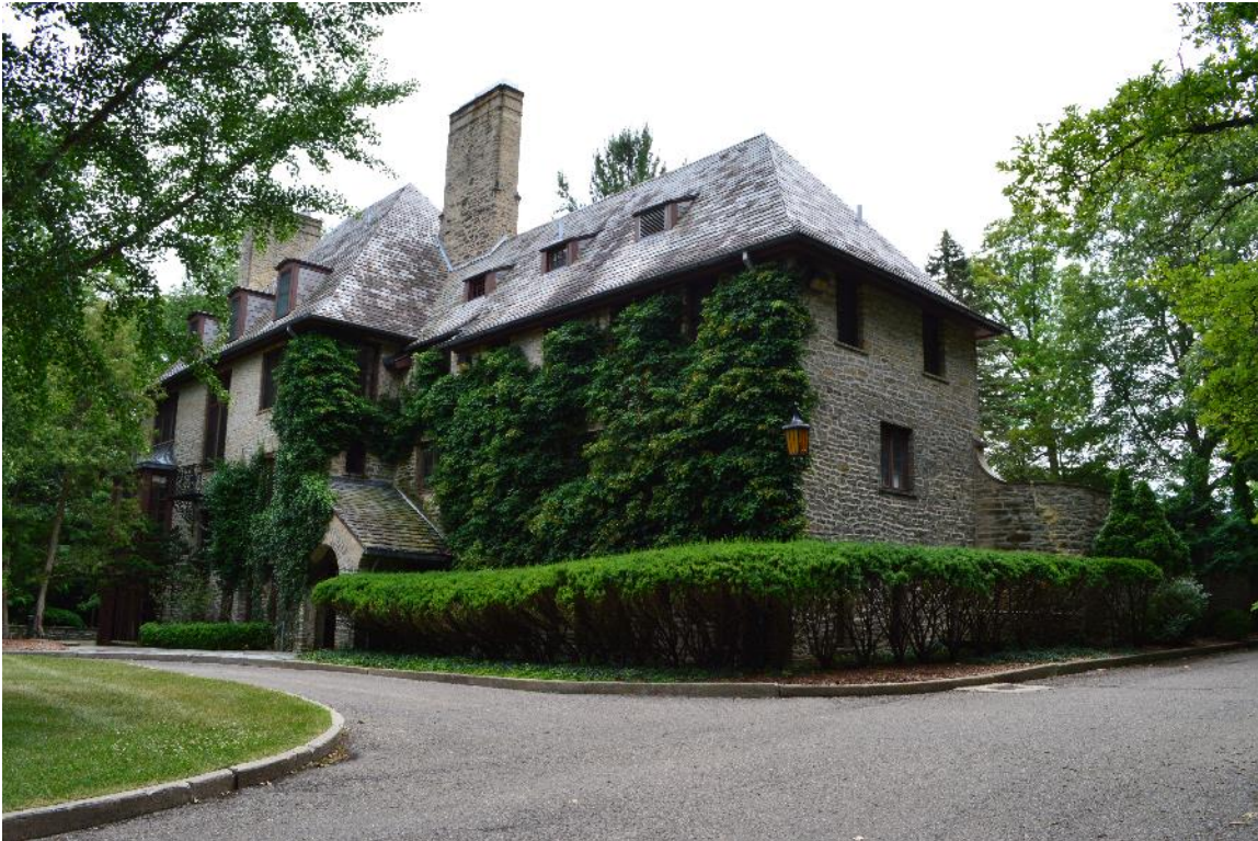
1 - Looking southeast at front of Inglis House and oval arrival court, July 2017
