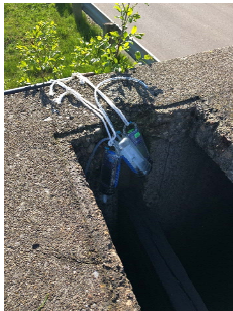
FIGURE 25: INFLUENT OVERFLOW STRUCTURE WITH MONITORS
