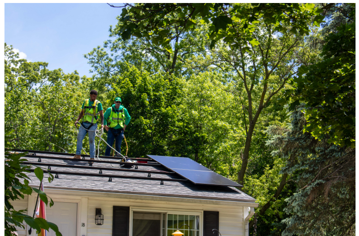
Solar Panel Installation in Bryant Neighborhood.
