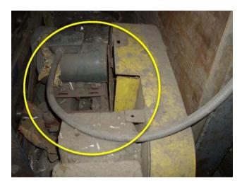
Power unit is filled with debris, replacement required.
