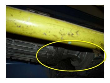
Gearmotor is leaking, replacement required.
