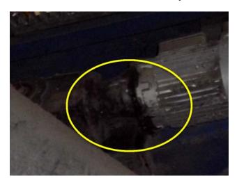
Gearmotor is leaking.
