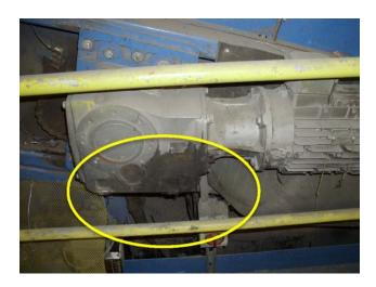
Gearboxes on all decks are leaking and needs to be replaced.
