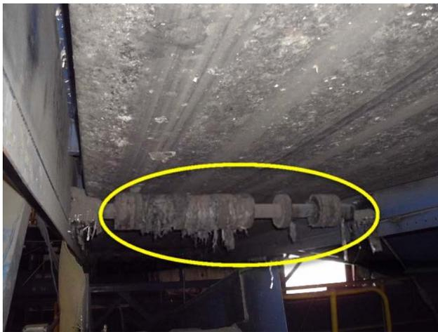
Return rollers are wrapped and worn, replacement required.
