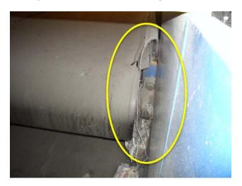
Belt is torn, debris is piled up under belt which is causing the tracking to be off and more strain on the belt.
