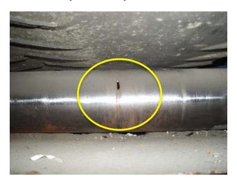
Return rollers are damaged. Replacement required.
