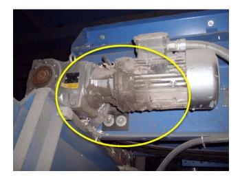
Gearmotor is leaking. Replacement required.
