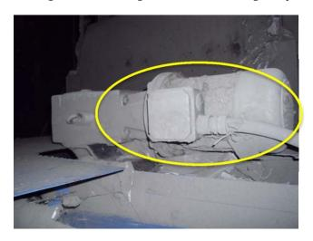
Motor is filled dust and surrounded by debris, replacement required.
