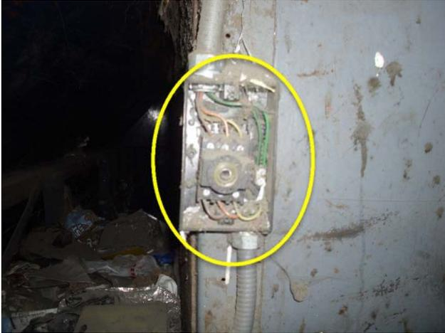
Cover has been removed from wiring. Unsafe exposure.
