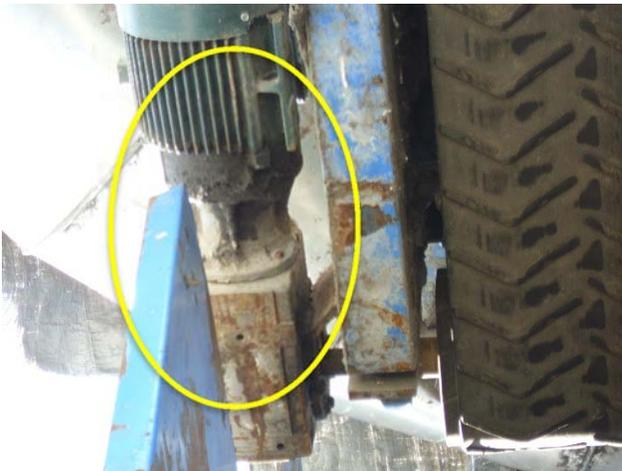
Gearmotor is leaking and needs to be replaced.
