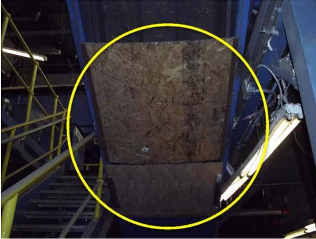
Plywood installed as belly pans, removal required.
