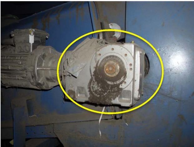
Gearmotor is leaking. It is held stable by zip ties. Replacement required.
