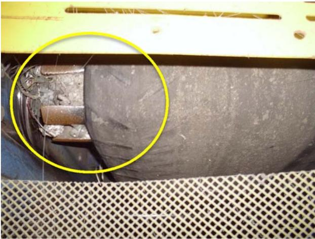
Pulleys are damaged, replacement of pulleys and bearings recommended. Belt tracking is to the right.
