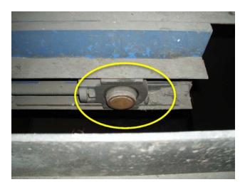
Bearings are worn, replacement required.
