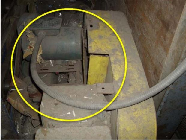
Power unit is filled with debris, replacement required.
