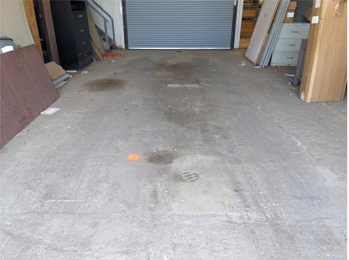
Image shows cleared boring location in orange and unknown utility marked in red crayon.
