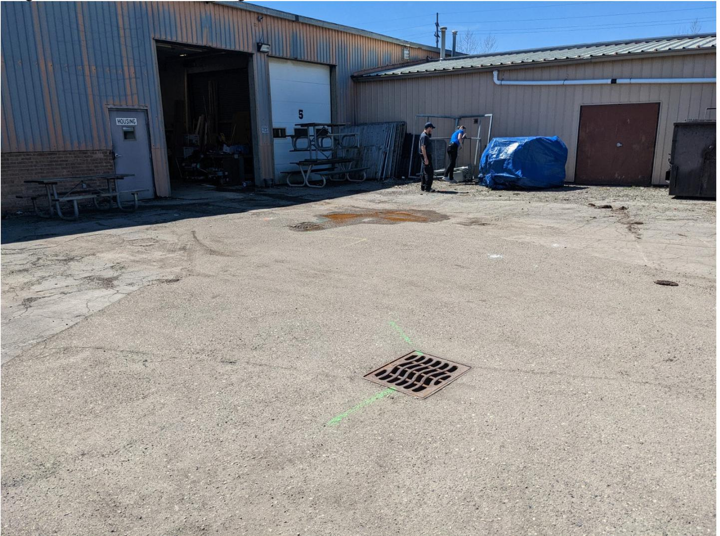
Image shows storm sewer marked in green and cleared boring location.
