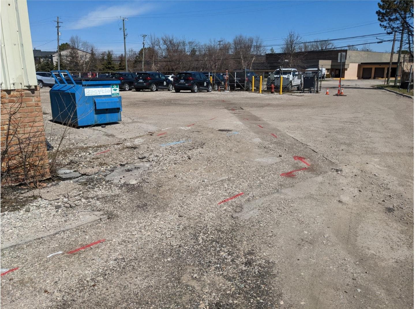
Image shows electric marked in red and water in blue.
