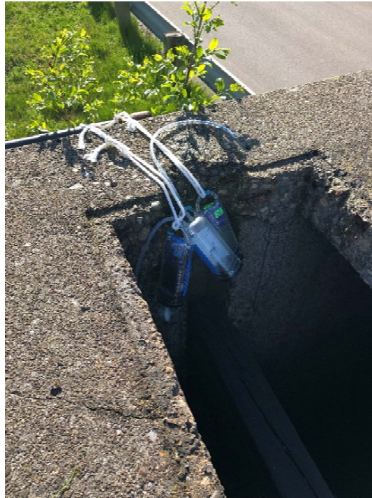
FIGURE 5: INFLUENT OVERFLOW STRUCTURE
