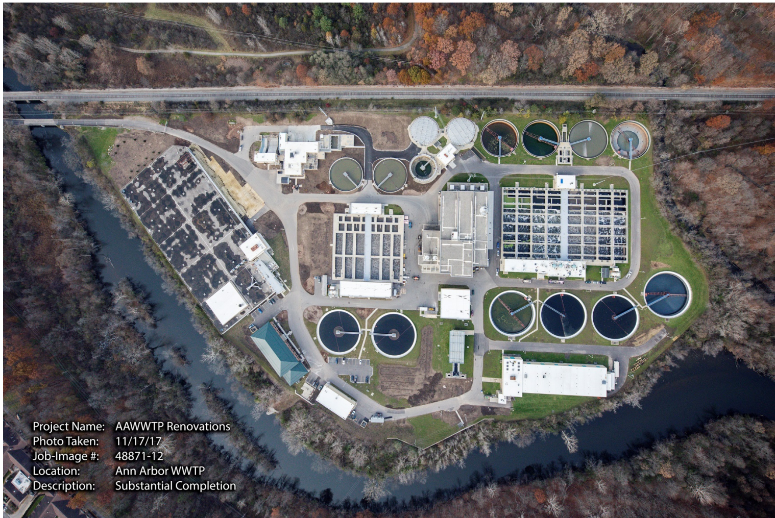
Figure 2-2. Plant Aerial View of Ann Arbor WWTP
