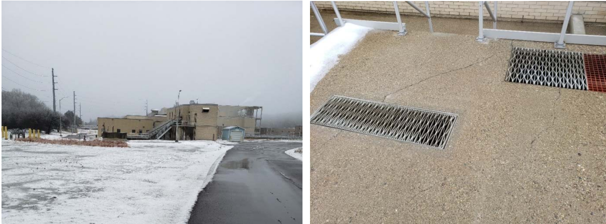
FIGURE 2: RAW SEWAGE LIFT STATION (LEFT) AND RISING WELL (RIGHT)
