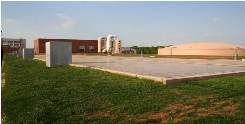
Figure 5-12. Photo of a Long-Life Media Biofilter System
