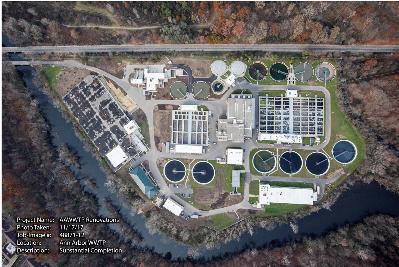
Figure 1-2. Plant Aerial View of WWTP
