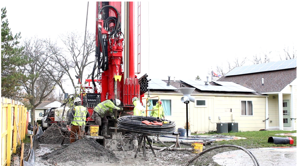
Drilling for the geothermal system at the Bryant Community Center.
