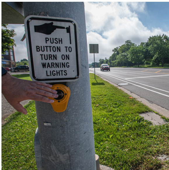
Accessible Pedestrian Signal
