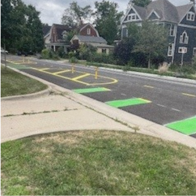
Fifth Ave. - Resurfacing
