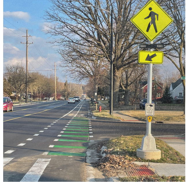
Platt Rd. - Resurfacing
