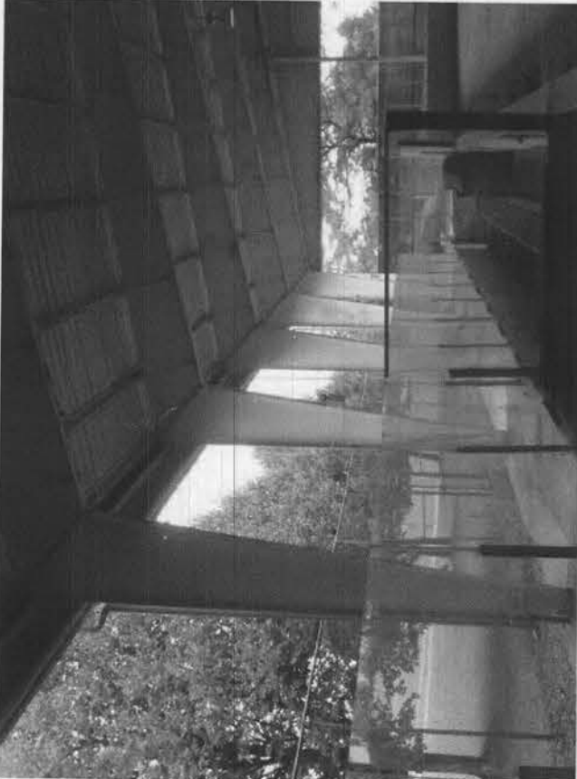
METAL ROOF DECK (TYPICAL)
