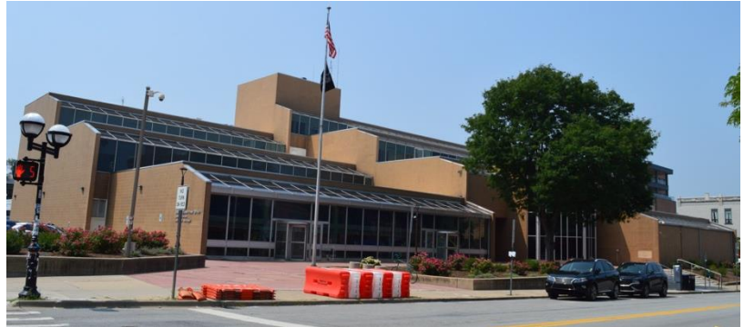
Photos 6 and 7 Looking Enoch House and Federal Building, July 2025
