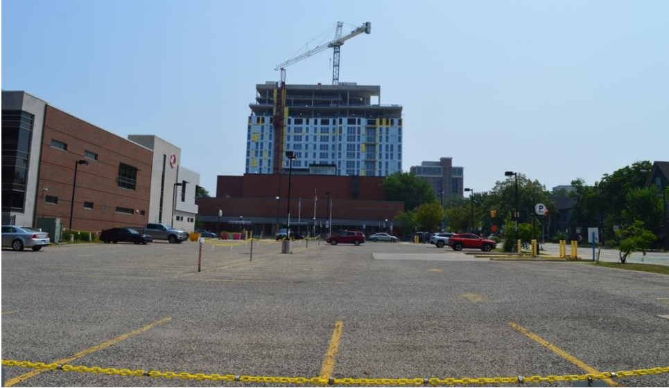
Photo 2 Looking east at project site, new building being constructed to the north, July 2025
