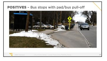
Another positive example is the bus stop along Pontiac Trail, with a bay to remove the bus from the active traffic lane, and concrete pad and shelter for transit users waiting for the next bus to arrive.
