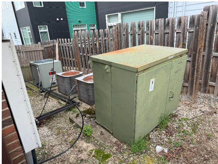
Photograph 5: Pad mounted transformer unit and exterior mechanicals area northeast of building.
