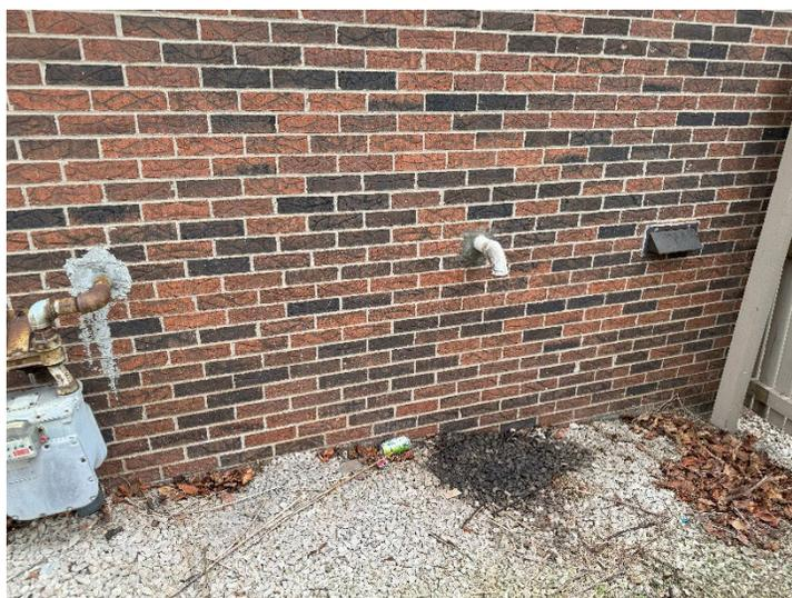
Photograph 6: Area of deminimis staining from compressor vent (northeast mechanicals area).
