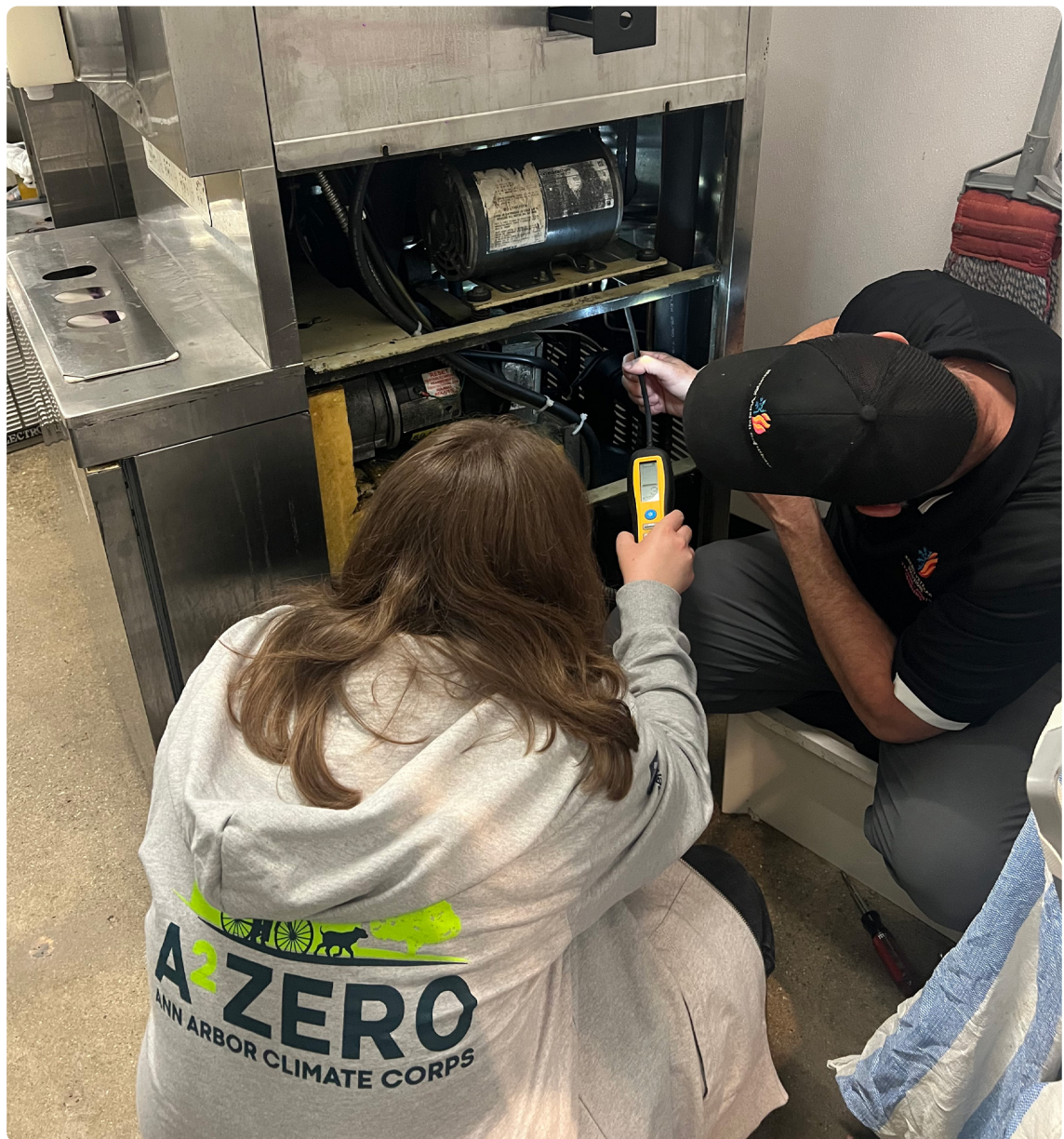
A refrigerant leak test at Bløm Meadworks.
