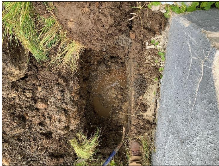
Photo 7: Plan View of Northeast Wall Corner: Saturated Soils and Local Erosion
