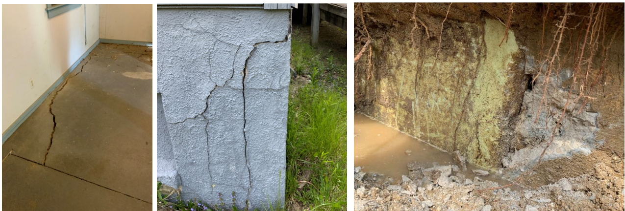
Foundation cracks and test pit filled with ground water, 2021.
