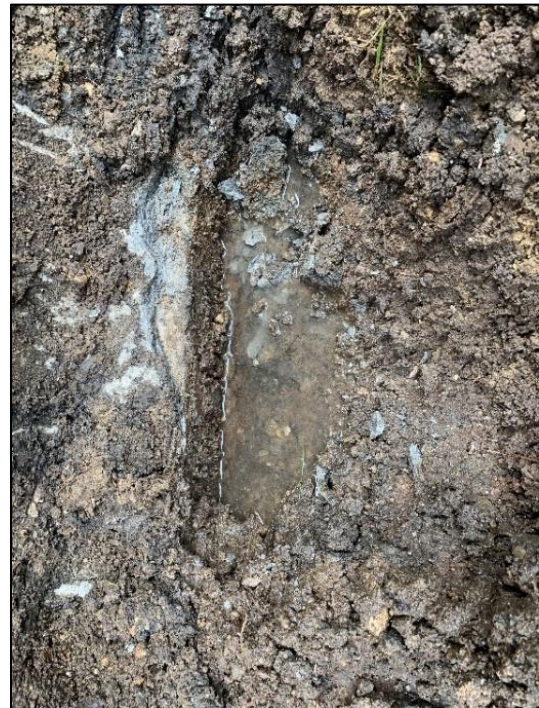
Photo 4: Saturated Top & Local Erosion Below Footing
