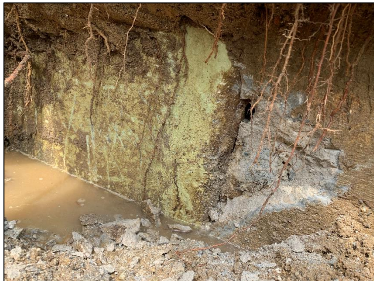
Photo 6: Damaged and Saturated Door Infill Area
