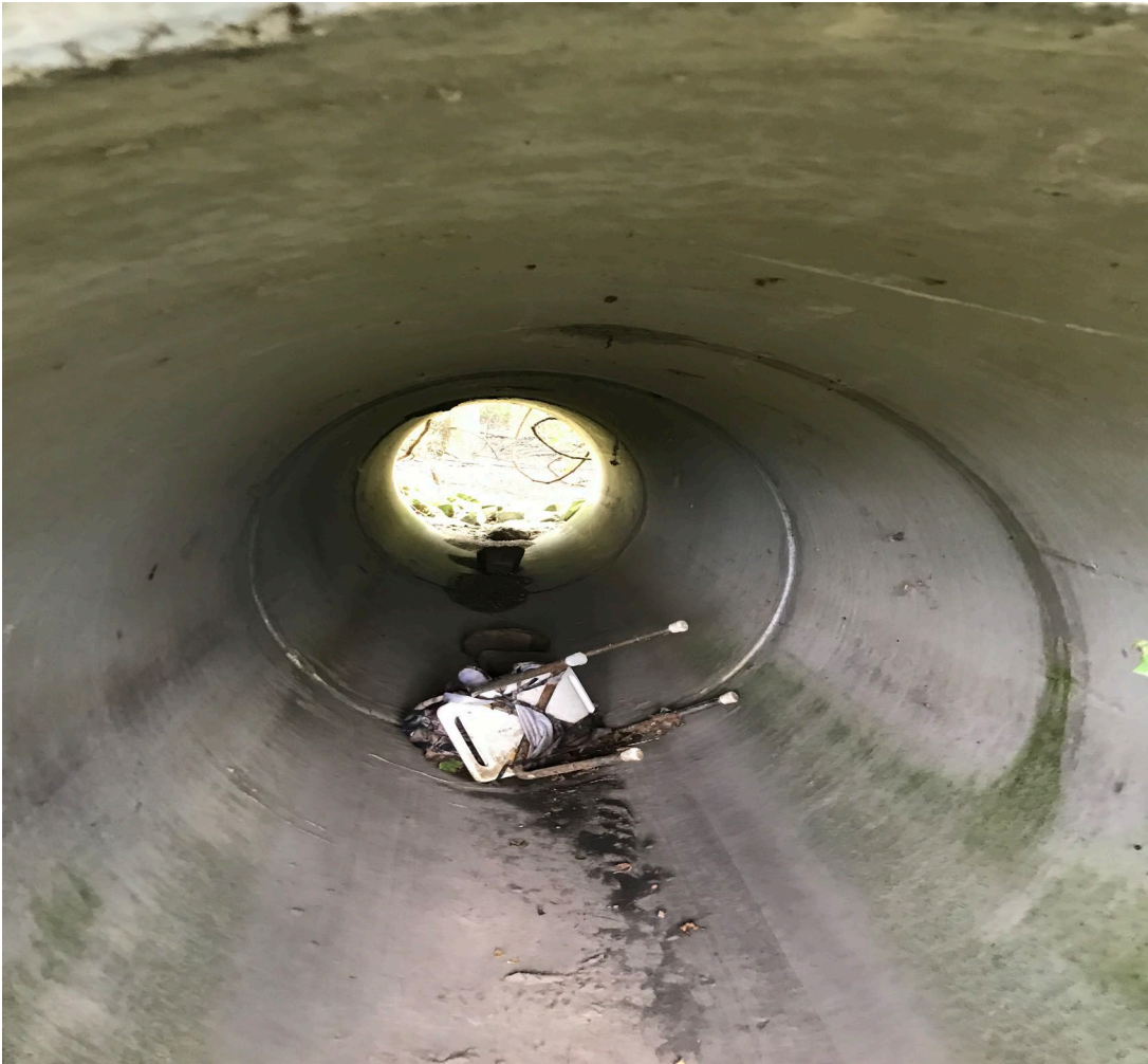
Figure 4. Four foot tall culvert leading off AOA into woods SW KARB
