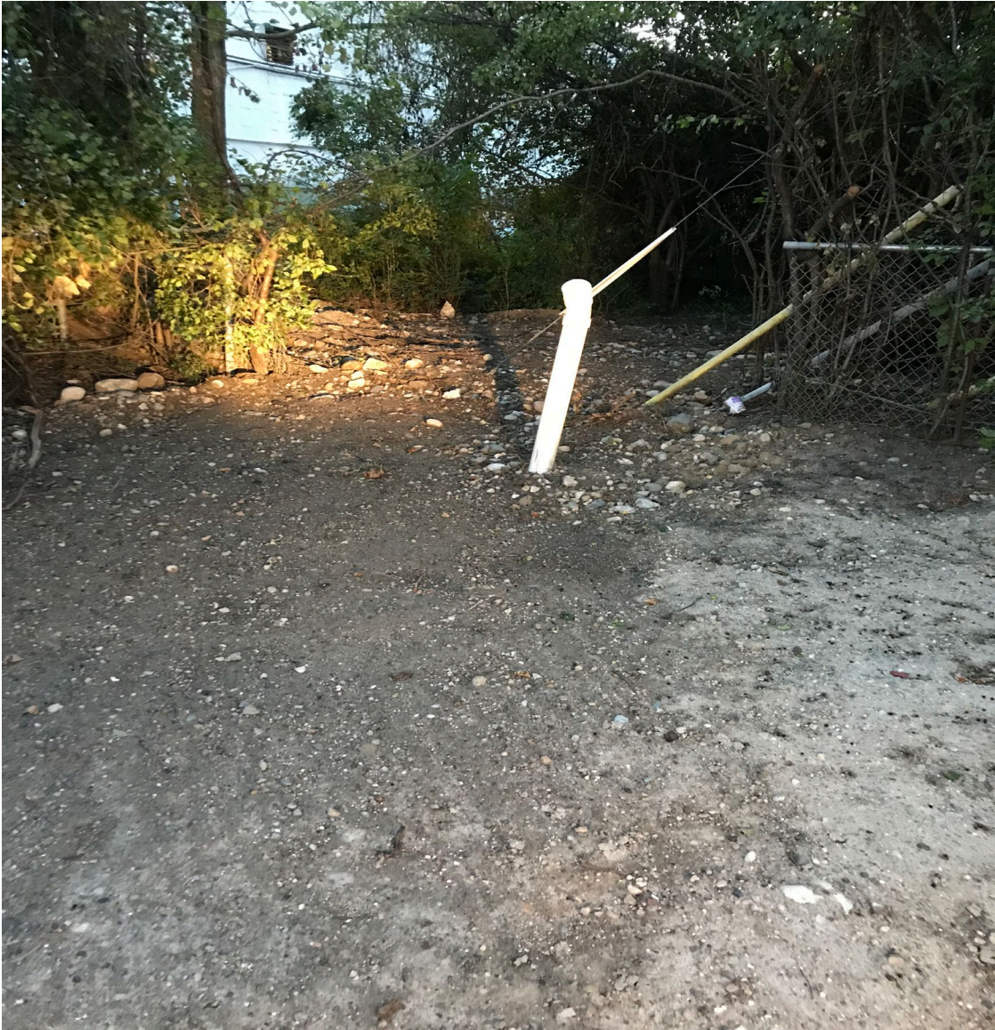
Figure 3. Open fence under construction NE KARB
