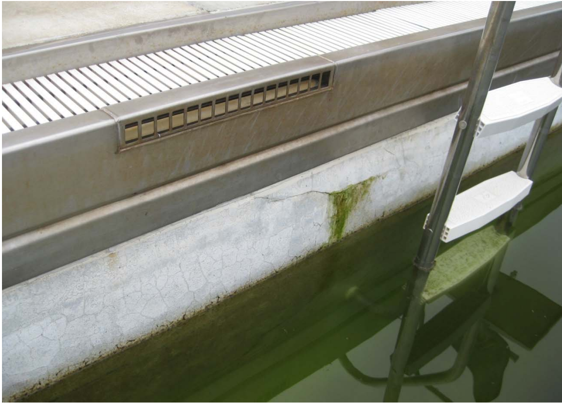
Condition of Marcite in deep pool
