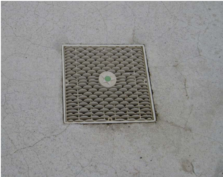
Grate in wading pool
