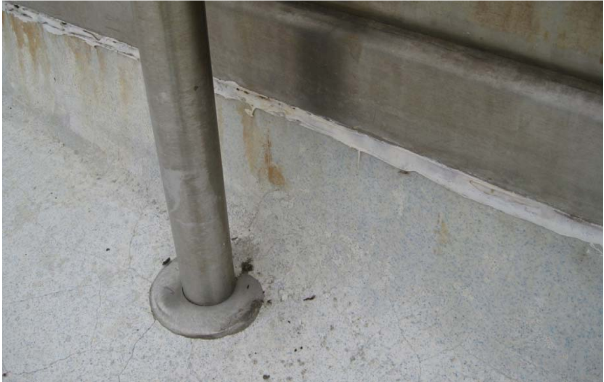
Install base cones on handrail system
