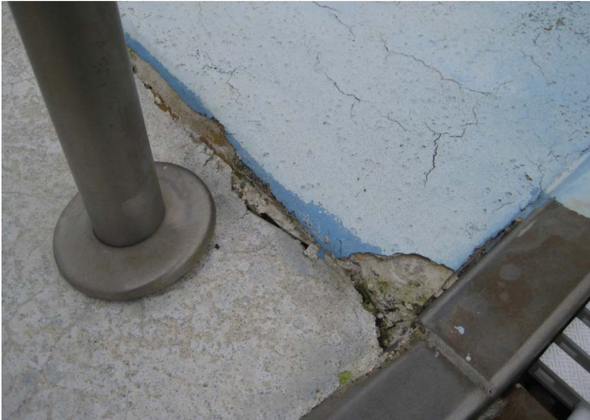
Spalling concrete
