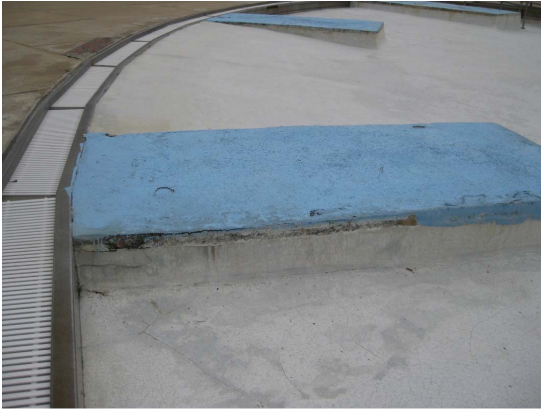
Concrete pads in wading pool
