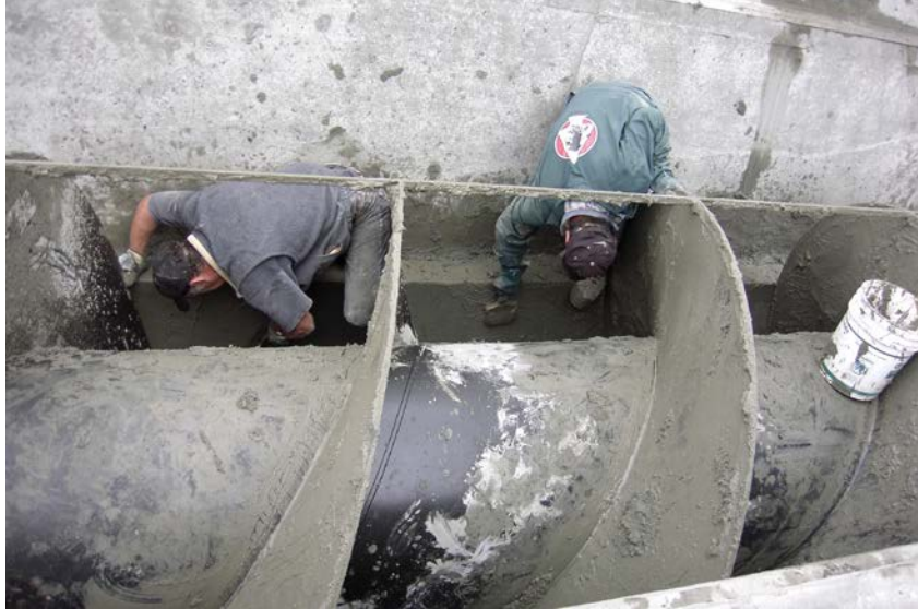
Hand Packing of grout:
