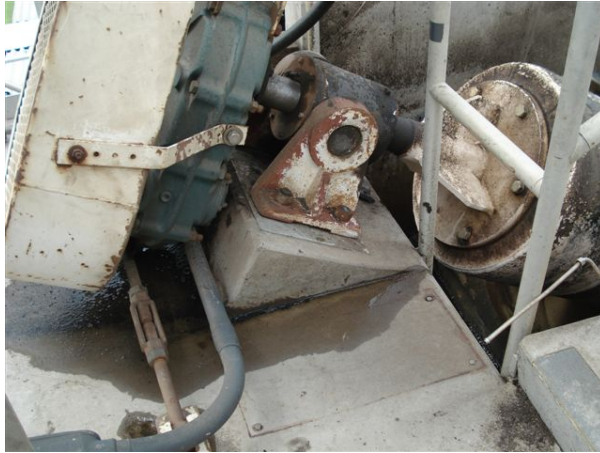
Upper bearing and concrete plinth to be demolished
