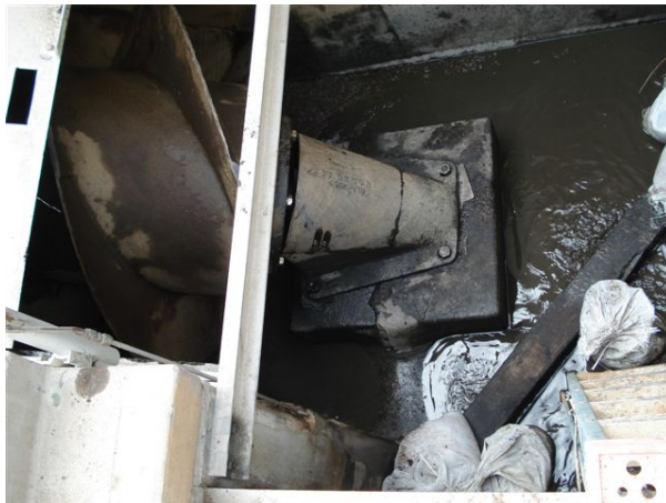
Lower bearing and concrete plinth to be demolished
