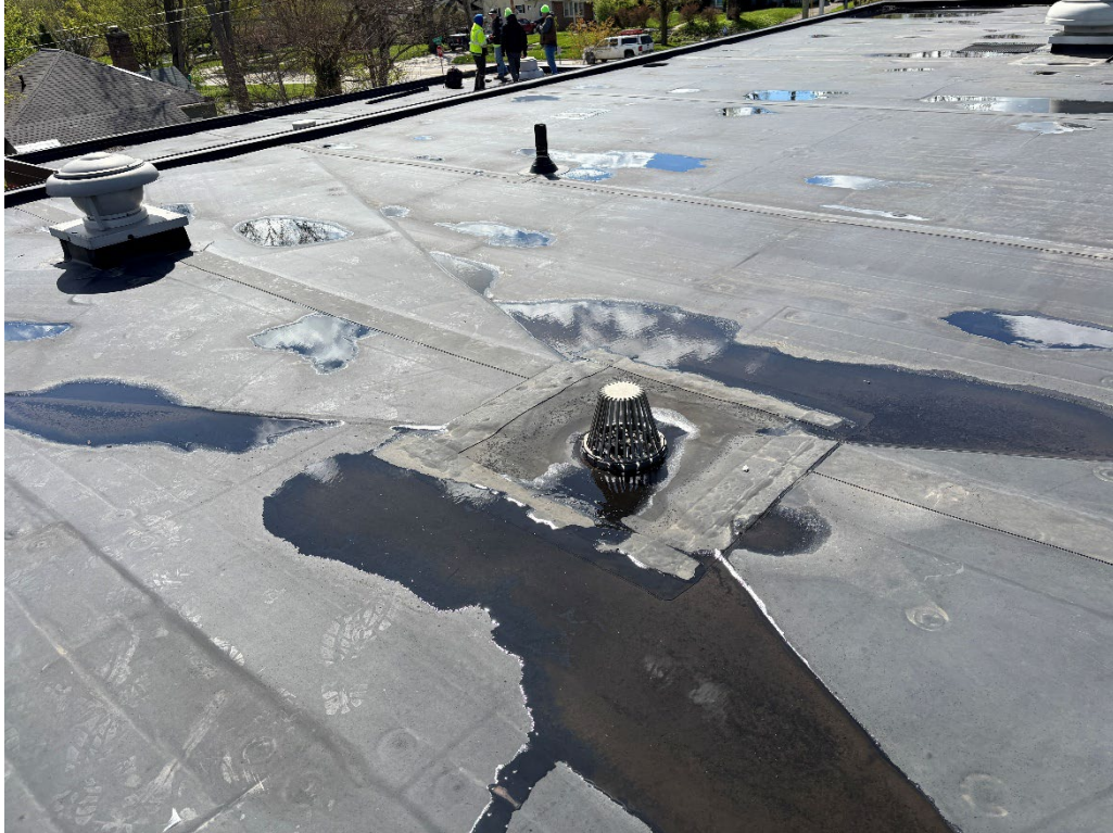
North Drain at Upper Roof
