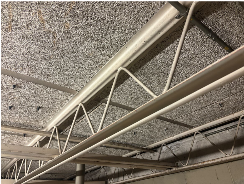
Existing Tectum Deck at Interior – Note Existing Fasteners to be Carefully Removed
