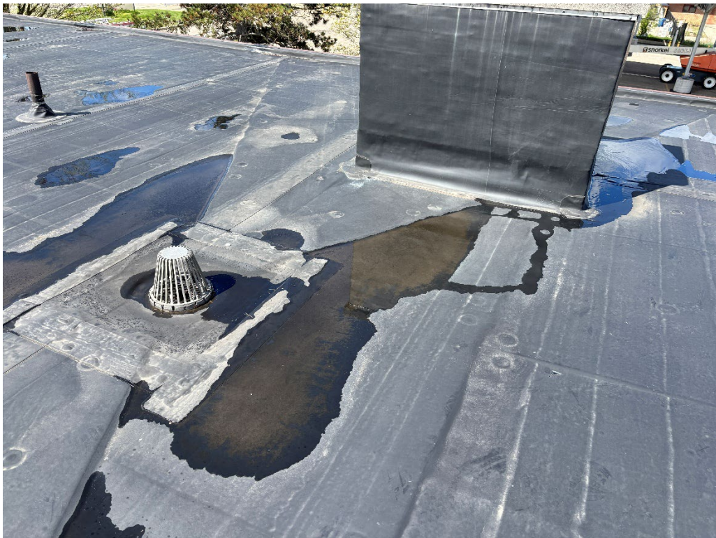
North Drain and Chimney at Upper Roof
