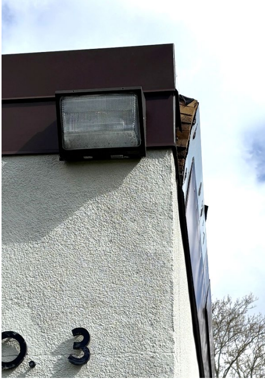
Leaning Section of Parapet at Southeast Side of Lower Roof To Be Addressed
