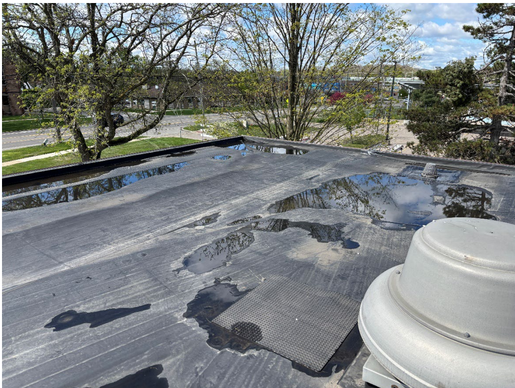
Southwest Corner of Upper Roof
